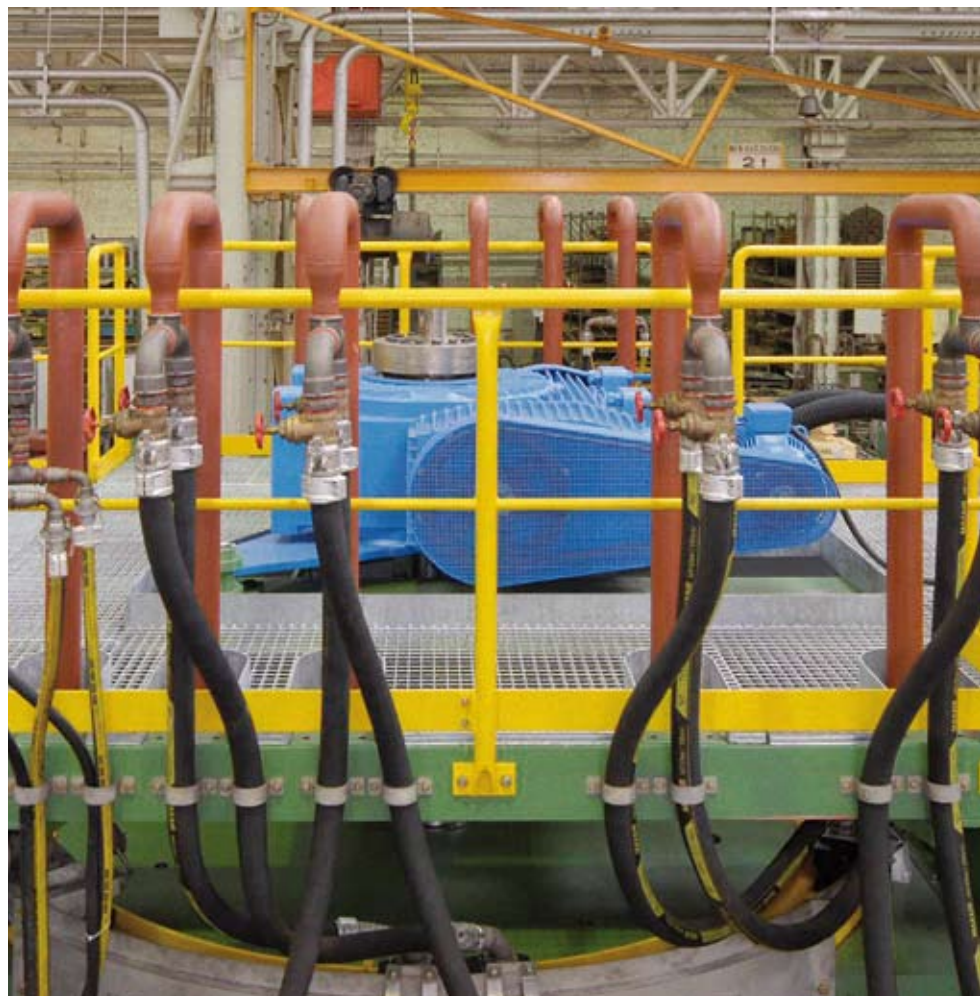
Assembly of the JONES WHIMS at MBE, Cologne
