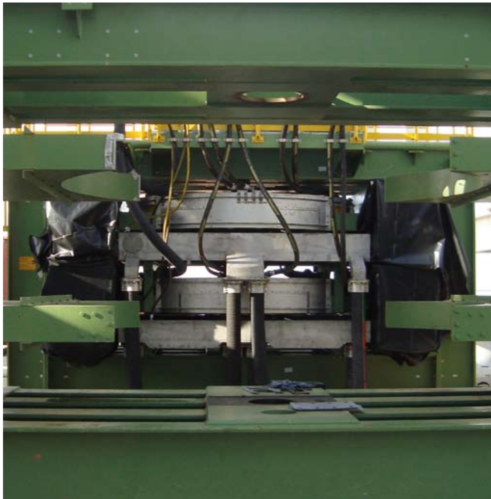
Installation of JONES at iron ore plant, Venezuela
